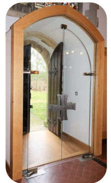
Internal transparent door at St Mary's, Balcombe
